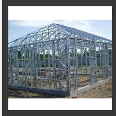
Heavy Steel Structure
